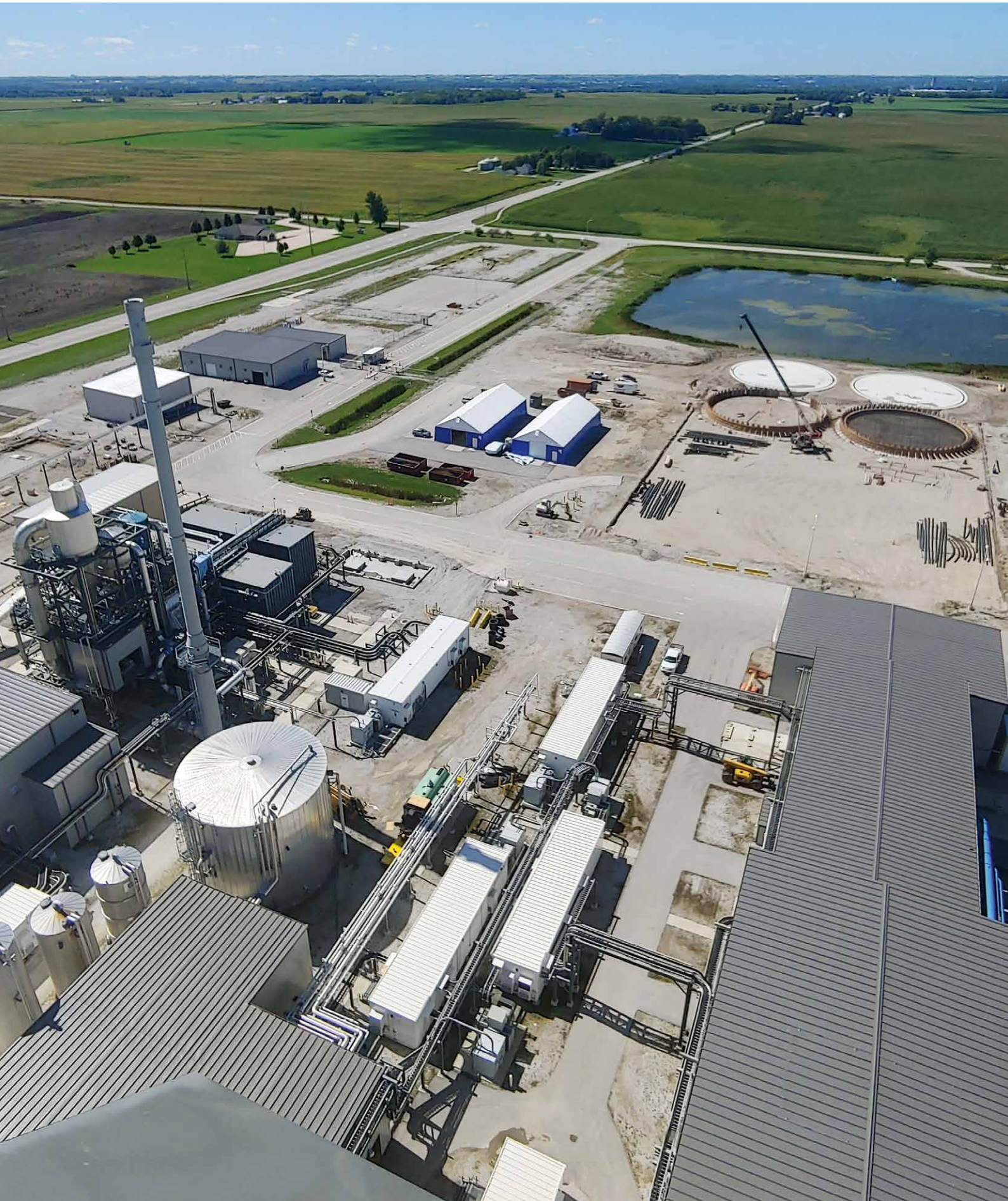
Under construction: Straw biomethane plant in Iowa, USA
