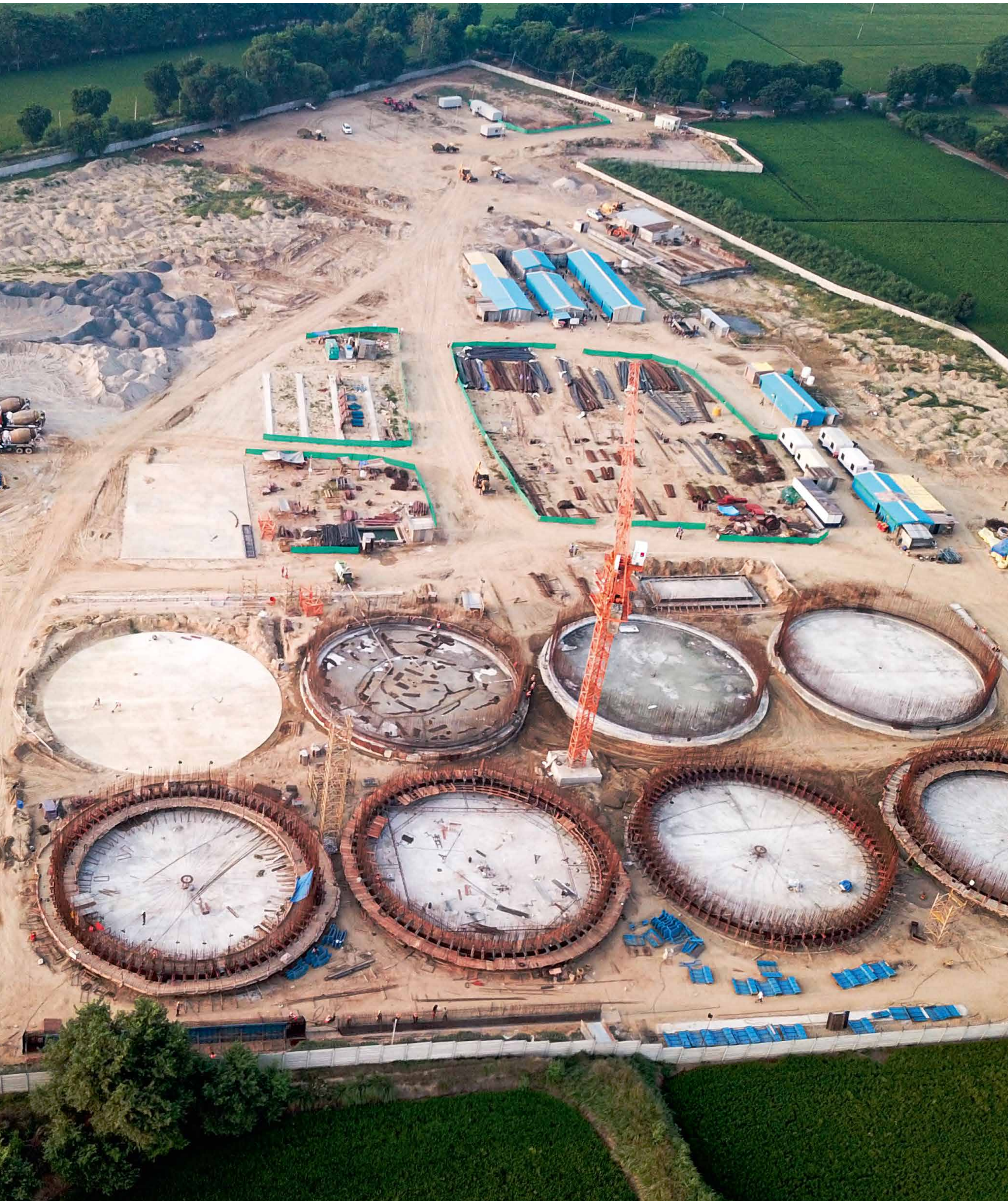
Under construction: Straw biomethane plant in India
