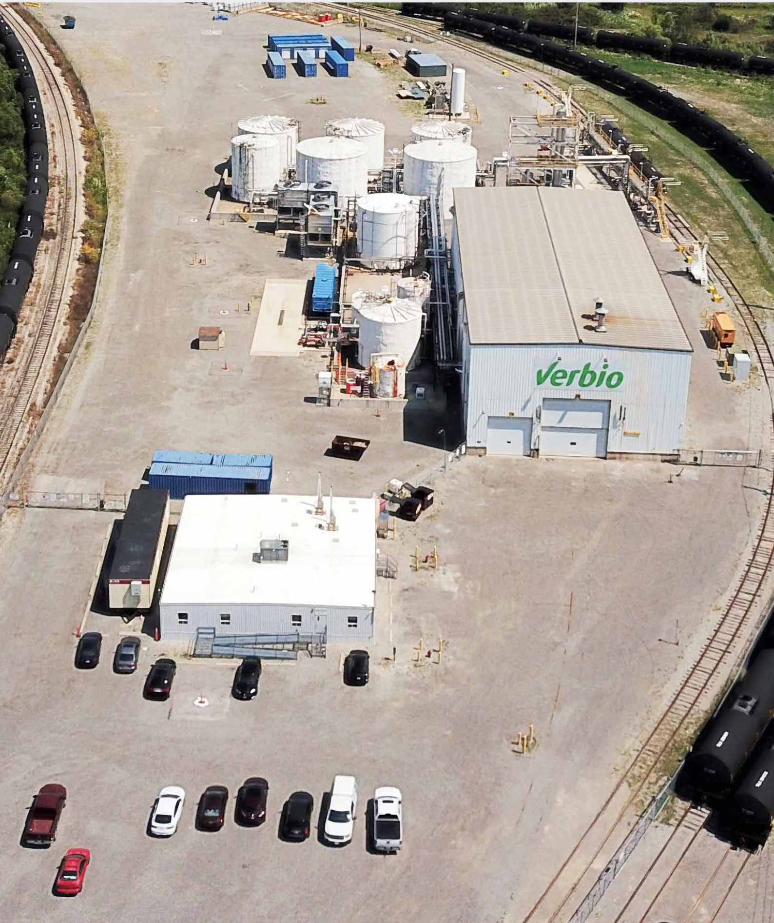
VERBIO-biodiesel plant in Welland, Ontario, Canada
